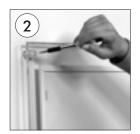
• Take off acrylic cover in the front. Mark the wall for mounting holes.
