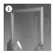
•Take off the yellow protection of the double sided tape along the sides of the frame and post it on the window.
